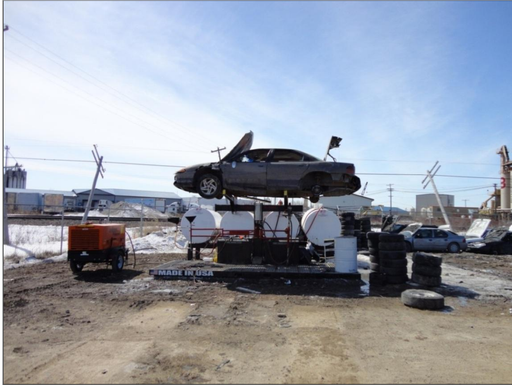
Figure 3: SEDA drain tower (fluid extraction system) located near the west perimeter of the site. Waste fluids are stored in the double-walled tanks behind the system.
